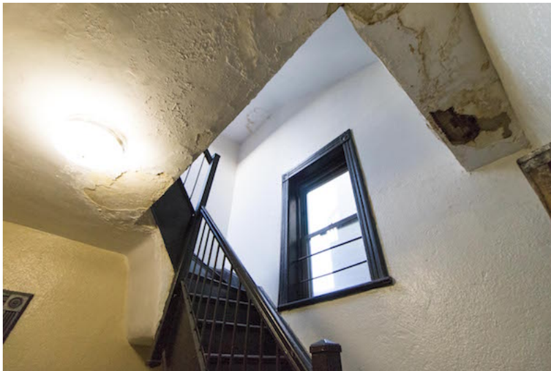
A leaky roof caused this water damage. Photo by Caleb Caldwell.
