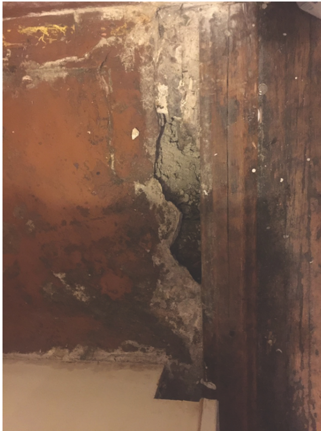
Crumbling drywall lets mice and roaches into the apartment. | Photo courtesy of a tenant
